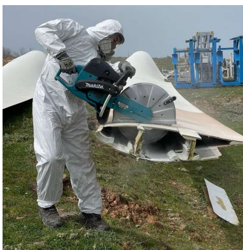
Figure 3: Blade cutting process
